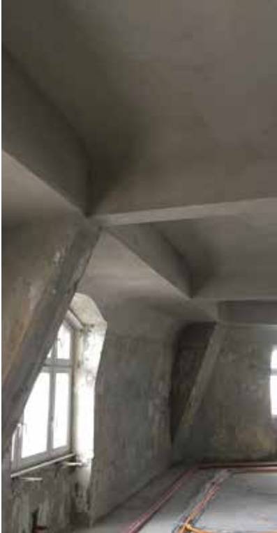
Ceiling and joists | felt-floated surface
