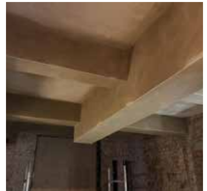
Ceiling beams with box protection
