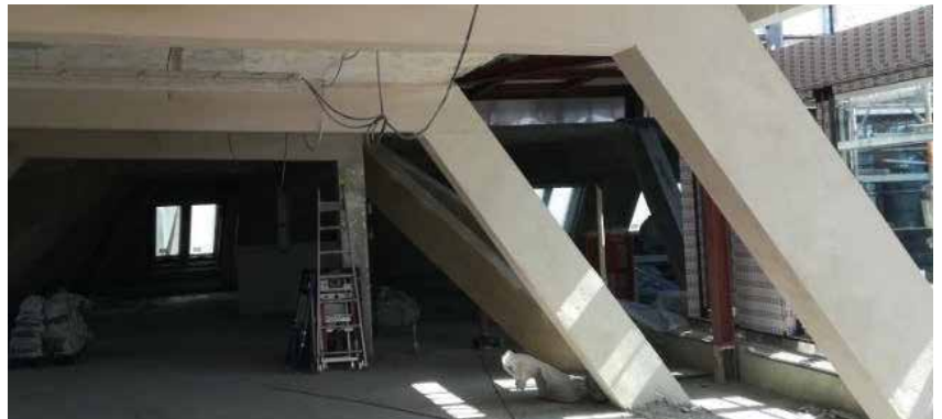
Steel structures as a design element
